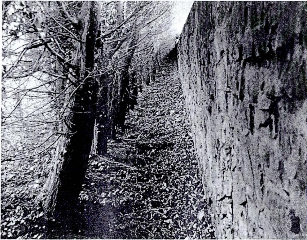
Fig 6 - Tree Group 5 (Leyland Cypress and Boundary Wall)
